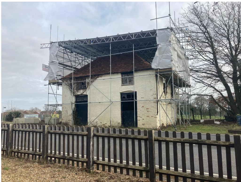
Plate 4. The Stable of the Bull Inn (List entry 1070807) fronting onto Ashford Road
