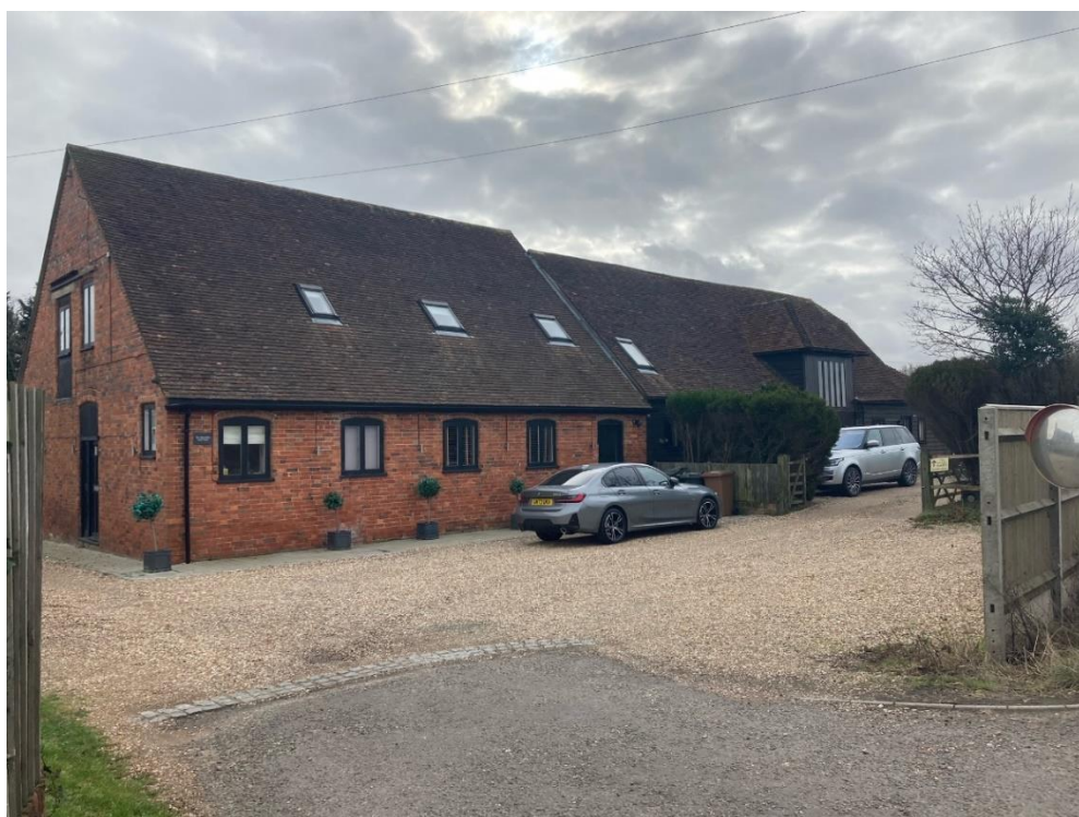
Plate 10. View of Weatherboarded Barn to south of Bridge farmhouse (List Entry 1362970) looking south-east
