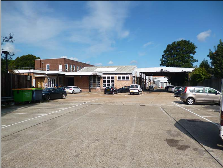
Plate 7. Former Charlton Green Sorting Office viewed from rear yard. Covered loading bay shown to the right. View facing north west.
