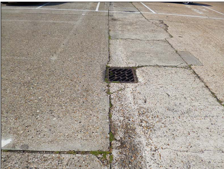
Plate 6. Drain cover in yard to south east of main building. View facing south east.
