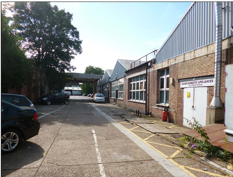
Plate 8. Rear of former Charlton Green Sorting Office showing retaining wall on the left. View facing south east.
