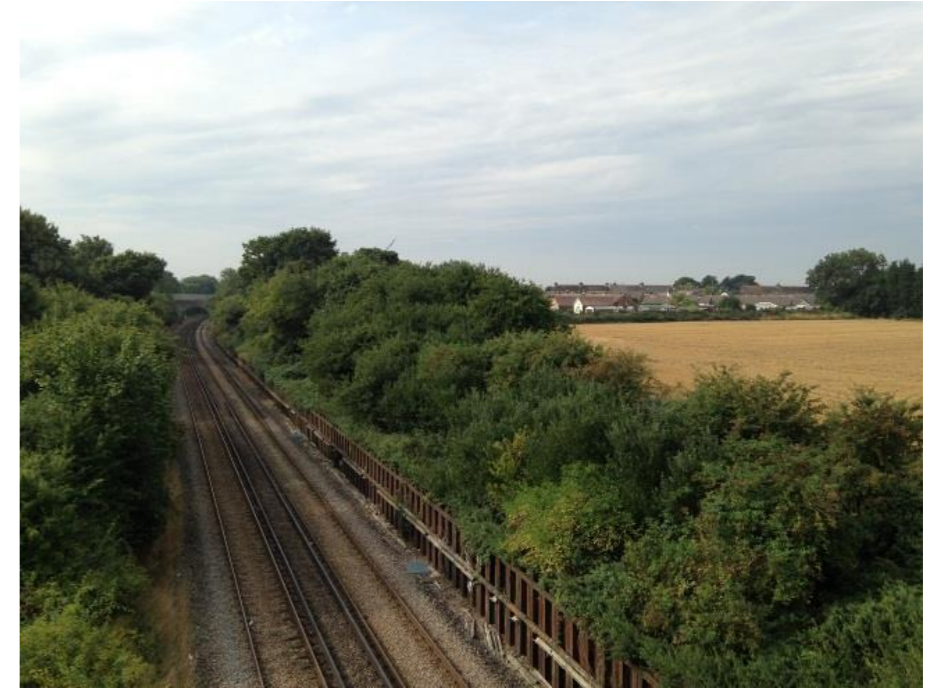
Figures 14: Railway along the eastern boundary of the site (the site is shown to the right of the image).
