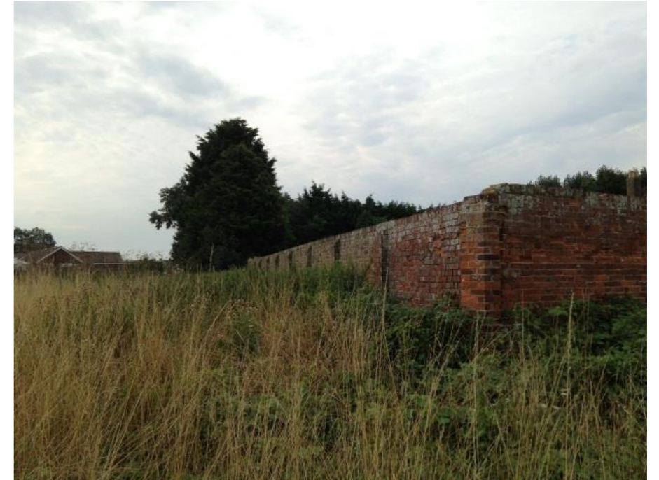
Figures 16: Garden wall at Great Grovehurst Farmhouse, at the south of the site.
