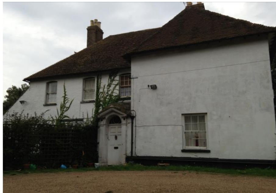
Figure 22: North façade of Great Grovehurst Farmhouse. Source: Site Visit (2013).
