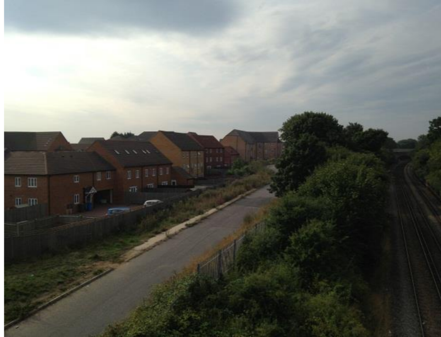
Figures 13: Railway and recent residential development to the east of the site. Source: Site Visit (2013).
