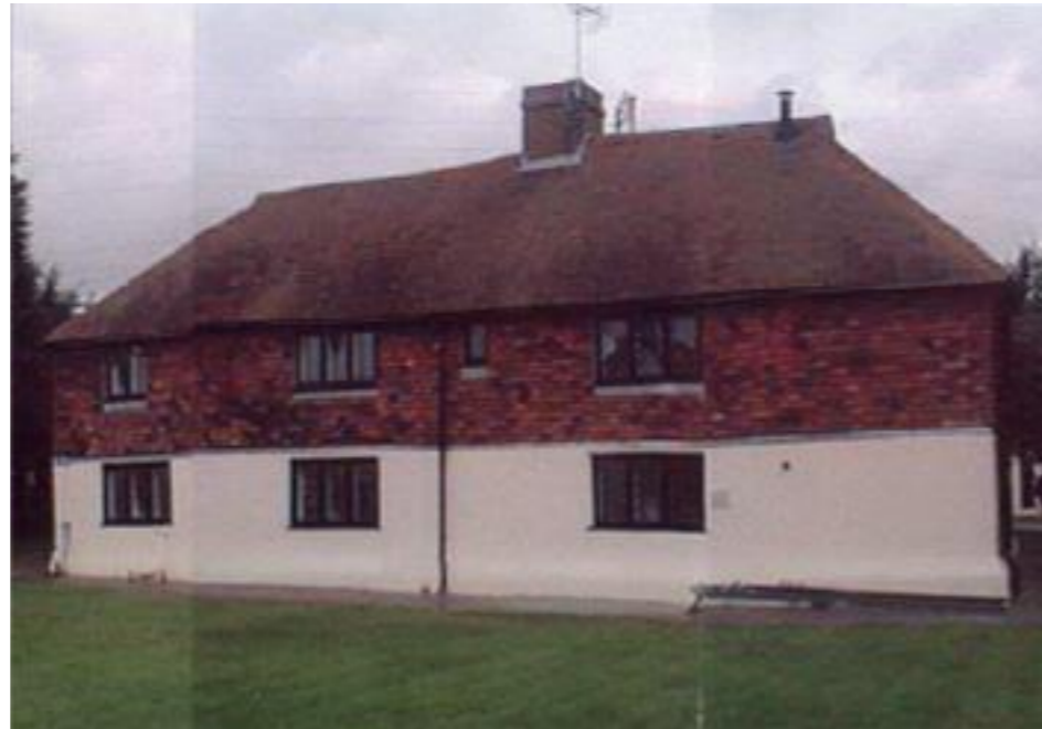
Figure 24: South western façade of Featherbed House. Source: Planning application SW/03/1337 at Swale Borough Council (2003).
