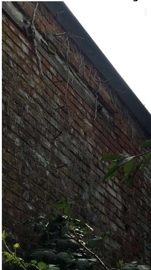
Photograph 10 – Root damage to garden wall bed joints.
