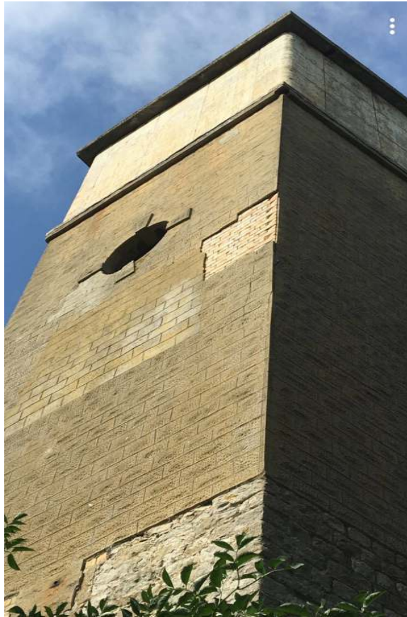
Photograph 5 – Water tower indicating de-bonded stucco render.
