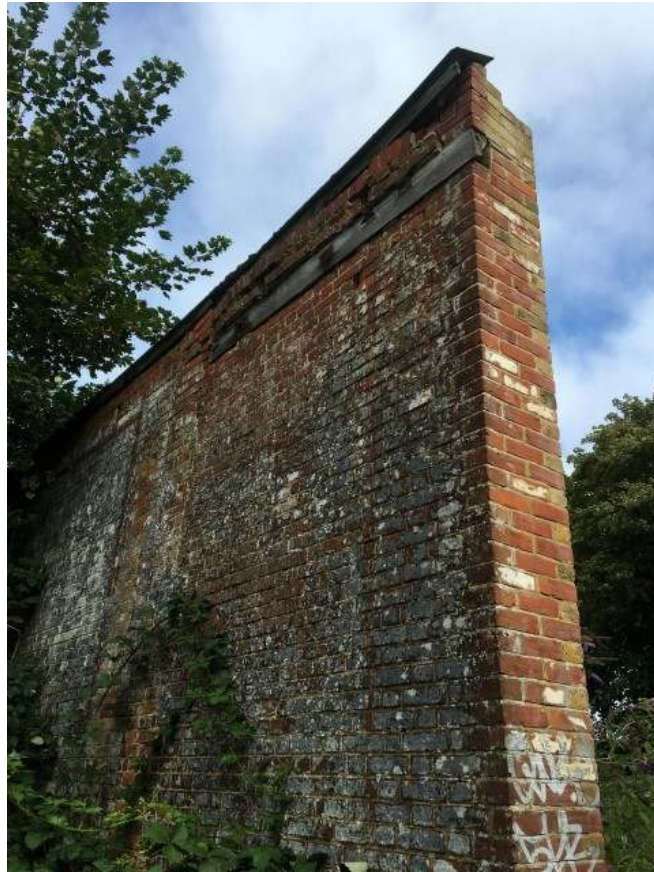
Photograph 9 – Garden wall with damage at the head.
