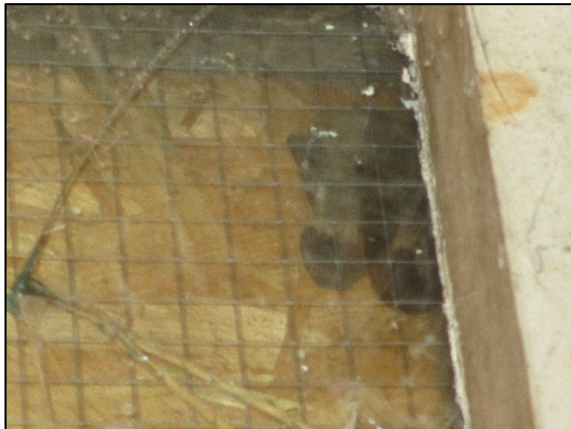
Photo 3 – Missing tiles on south 'stables' section of B11
