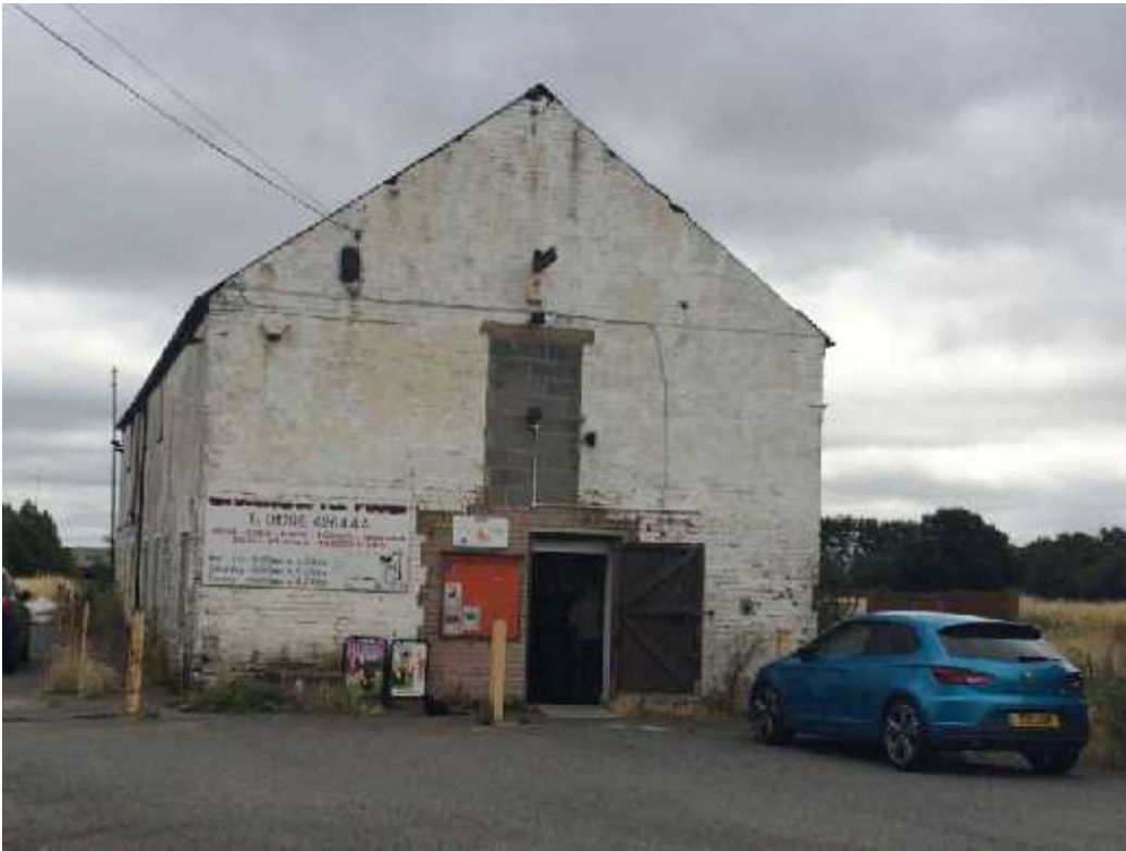
Plate 7 – West facing elevation of Building 4
