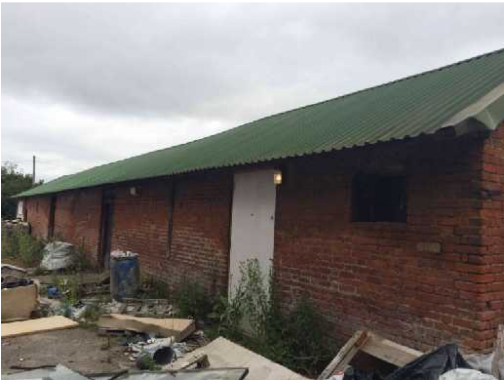
Plate 11 – External view of Building 5. Possible bat access points shown in red
