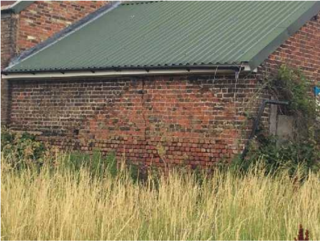
Plate 9 – Large crack in the brick wall at the south east of Building 4
