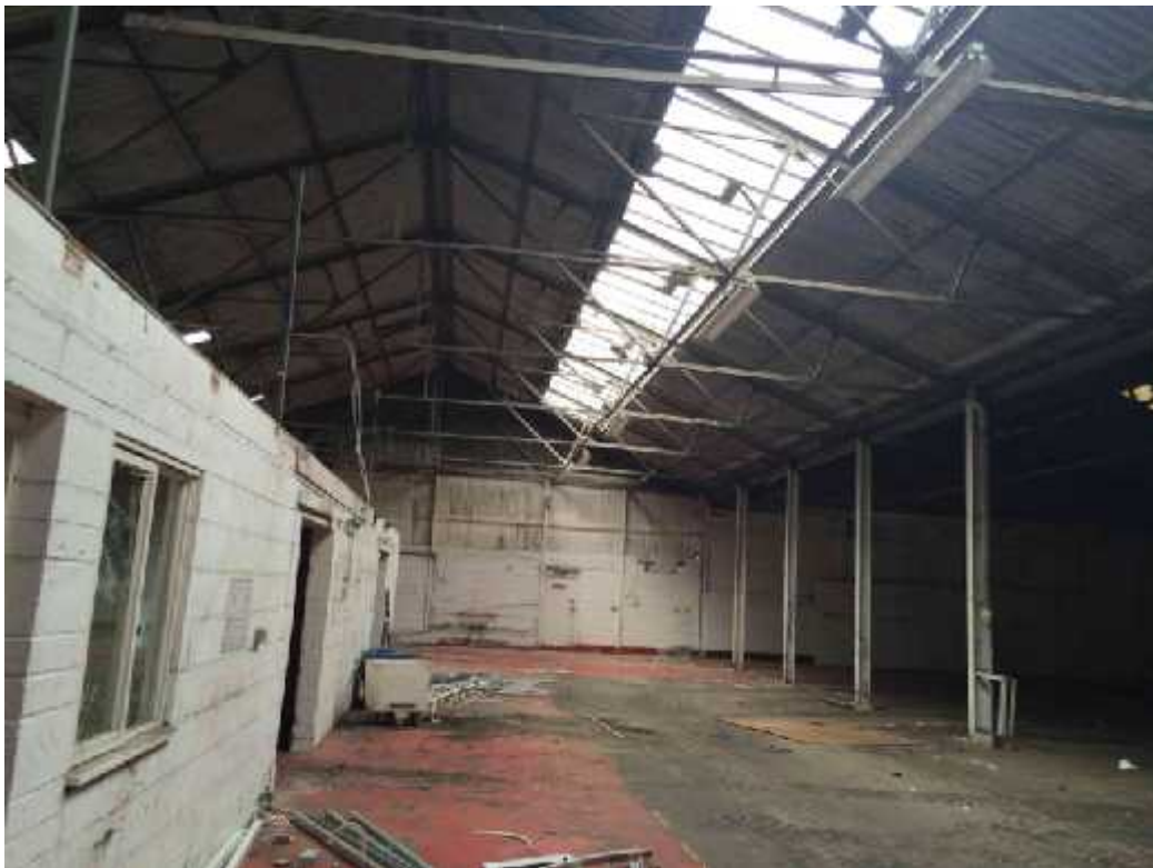
Plate 6 – Internal view of Building 3
