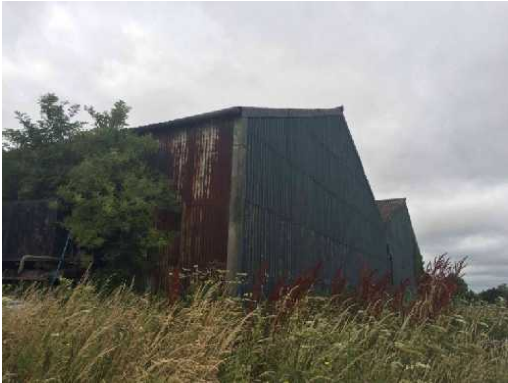
Plate 5 – External view of Building 3
