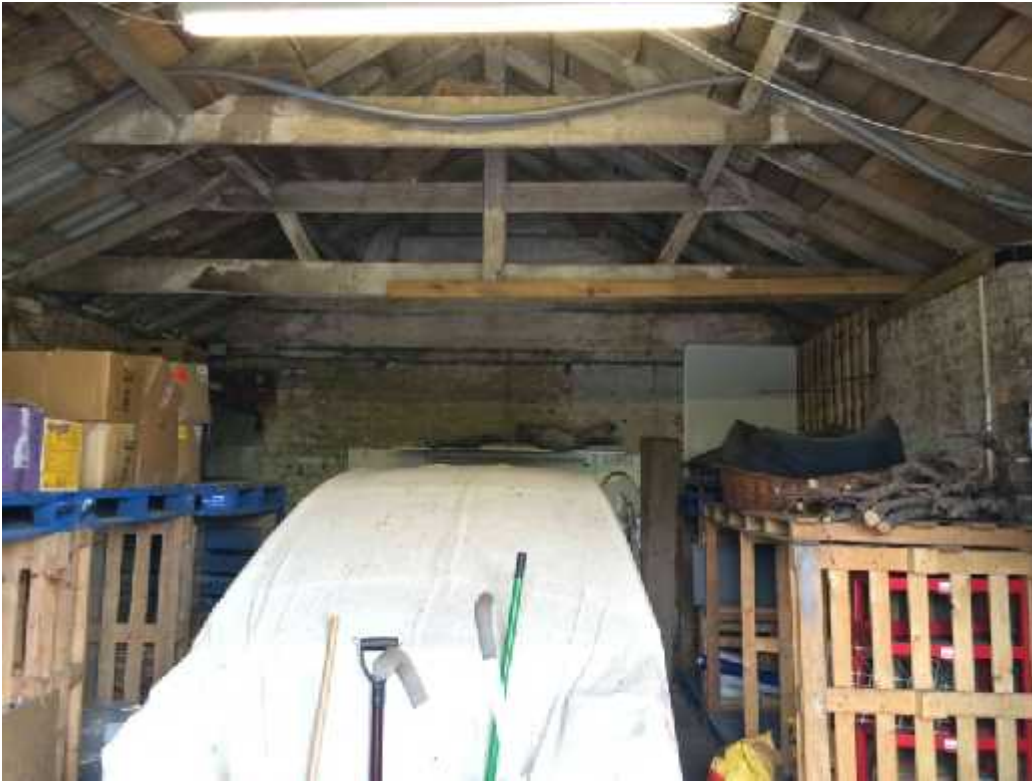
Plate 12 – Internal view of the western stable section of Building 5. Timber boards at the internal gable ends and timber roof lining have potential for crevice dwelling bats, and the internal space has potential for void dwelling bats
