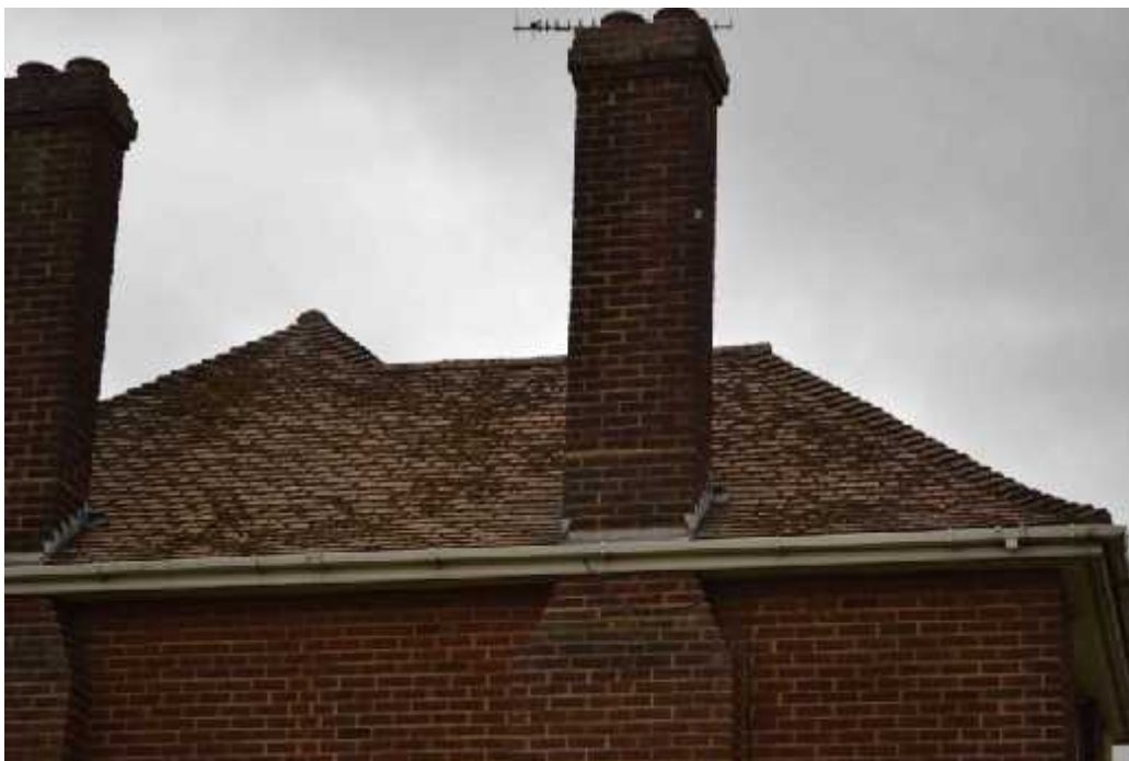
Plate 2 – North facing view of Building 1, showing gap beneath the central ridge tile, which is an example of one of the potential bat roost/access features within the building
