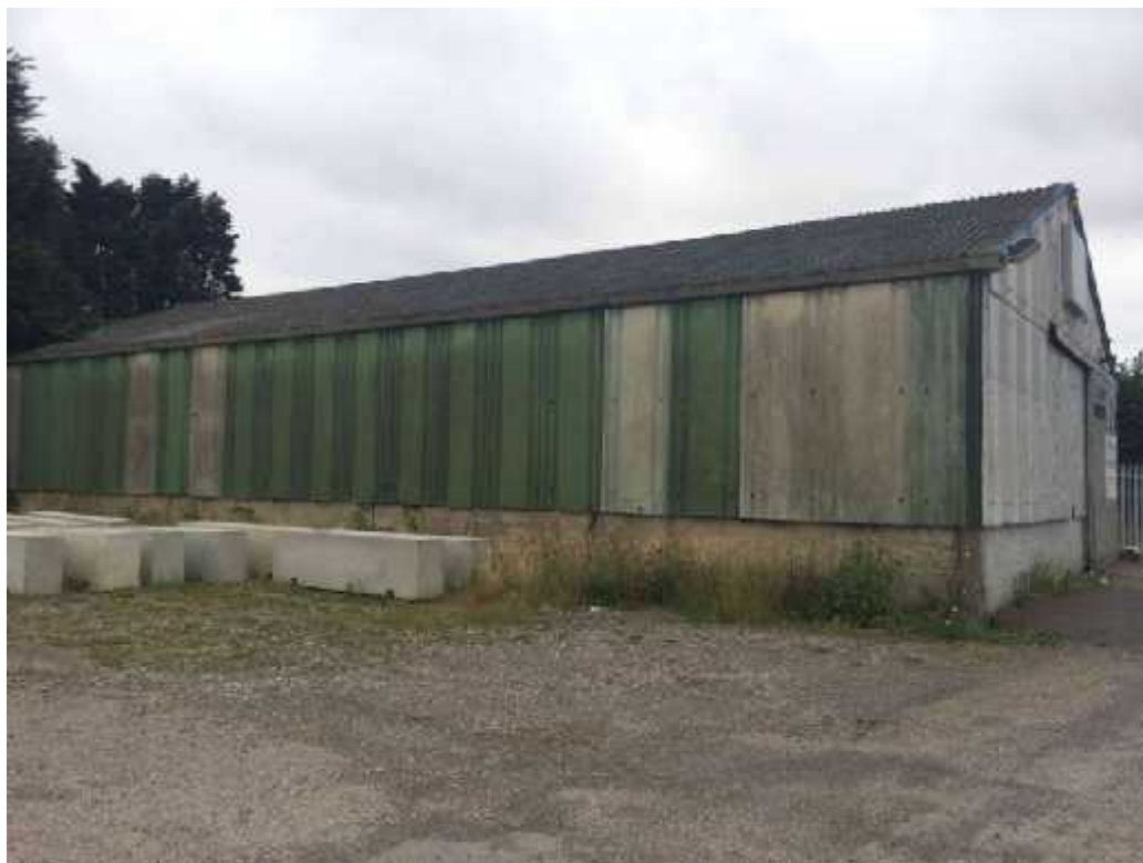
Plate 4 – External view of Building 2
