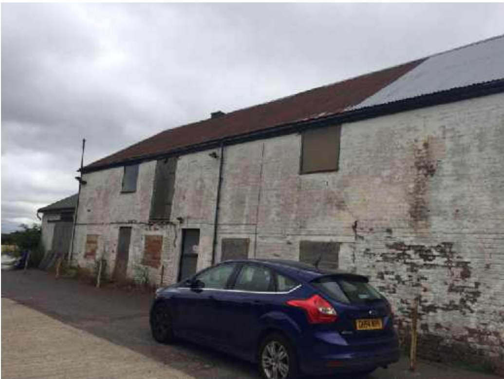
Plate 8 – North facing elevation of Building 4 showing gaps in wooden door allow potential bat access
