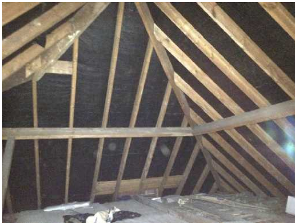
Plate 3 – Internal view of the roof void, showing lining in a good condition
