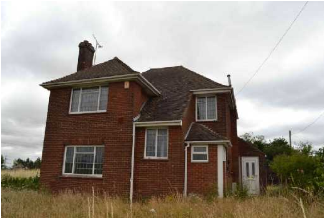
Plate 1 –East facing elevation of Building 1
