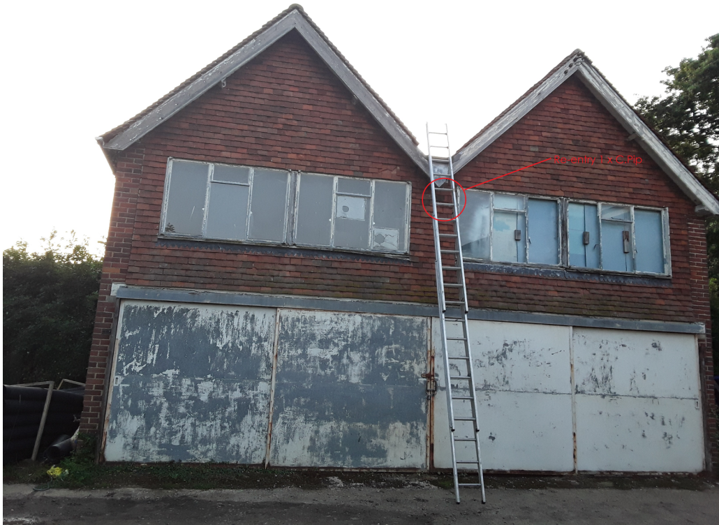
Figure 4: Western elevation of No. 5 with roost location
