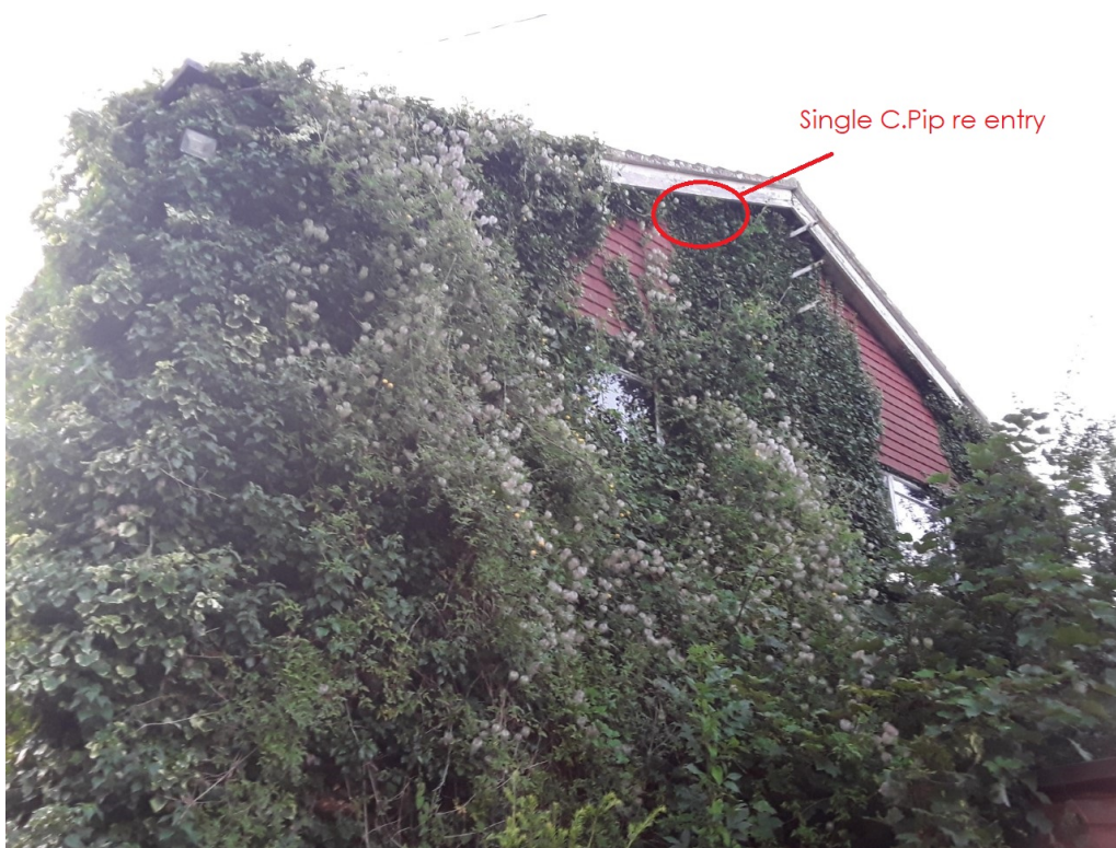
Figure 3: Western elevation of No. 3 with roost location
