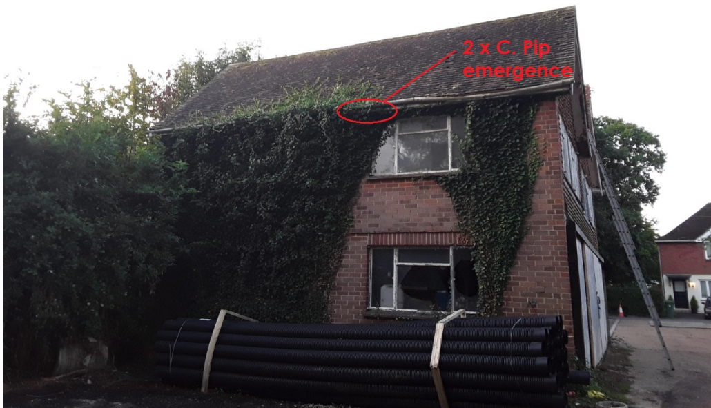
Figure 5: Northern elevation of No. 5 with roost location
