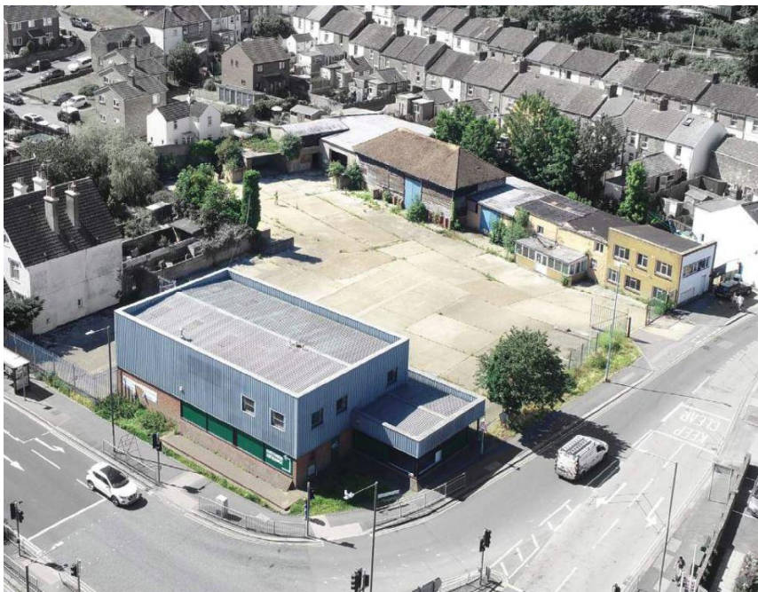
AP 1. The site (looking south)
