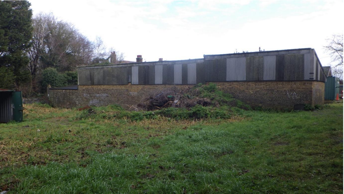
Plate 13: Building abutting the cattle shed/barn, looking north-east
