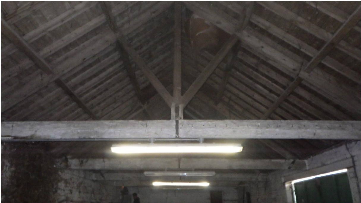
Plate 11: Interior of cattle shed/barn roof, looking west
