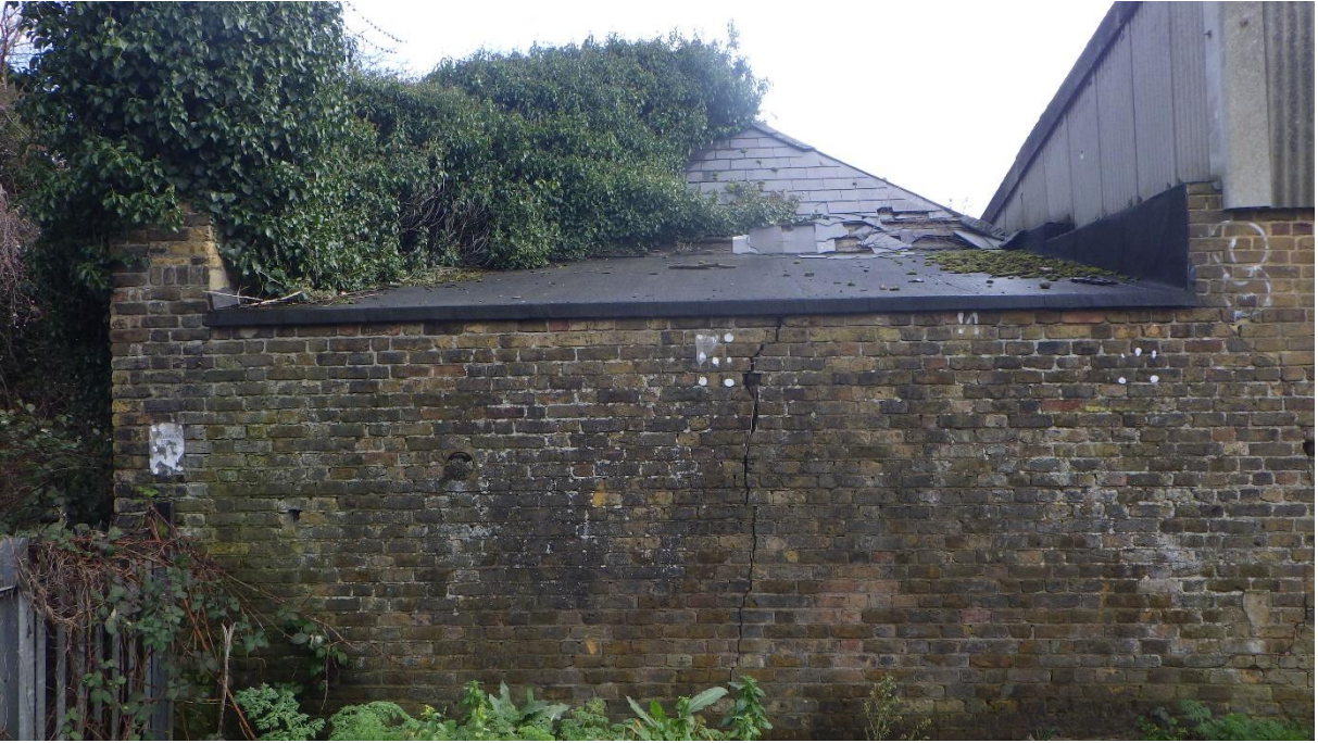
Plate 5: The west end of the cattle shed/barn, looking east
