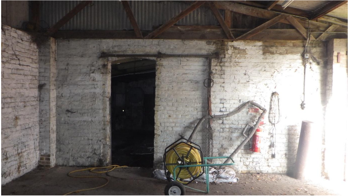
Plate 7: The west end of the cattle shed/barn (extension), looking north
