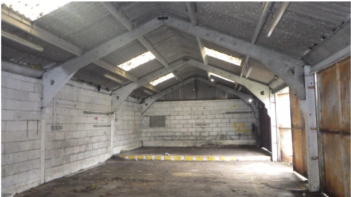
Plate 20: Interior of agricultural building at east of Ste, looking south
