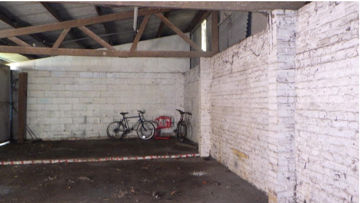
Plate 14: Building abutting cattle shed/barn, interior (north end)
