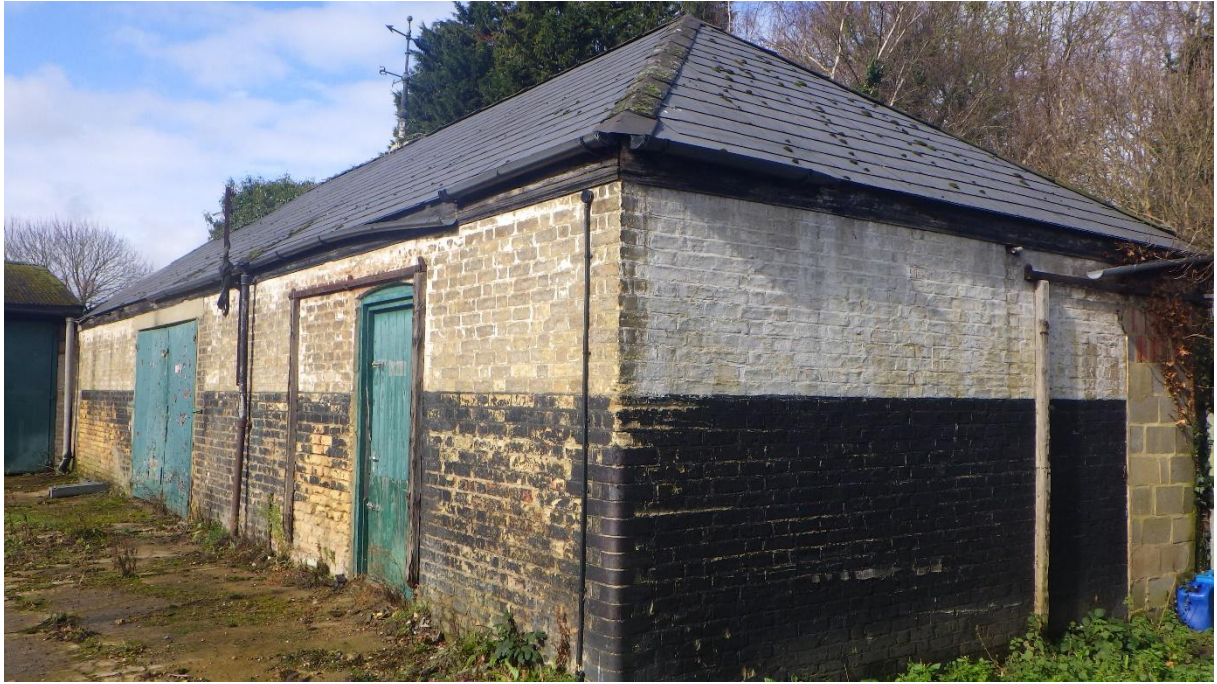
Plate 3: The cattle shed/barn, looking north-west
