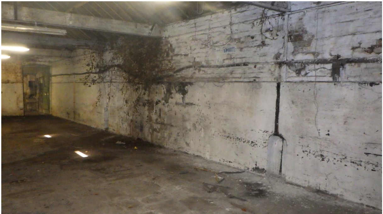
Plate 10: Interior of cattle shed/barn, looking north-west
