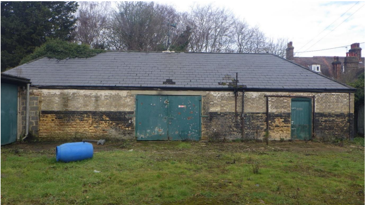
Plate 2: The brick cattle shed/barn, looking north
