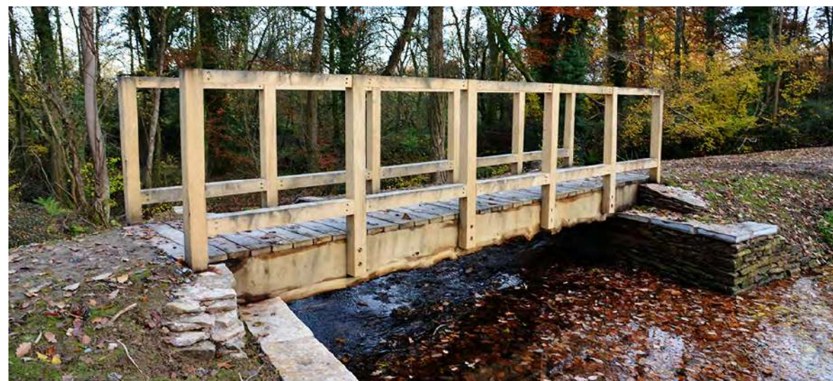
Timber bridge over Iwade Stream
