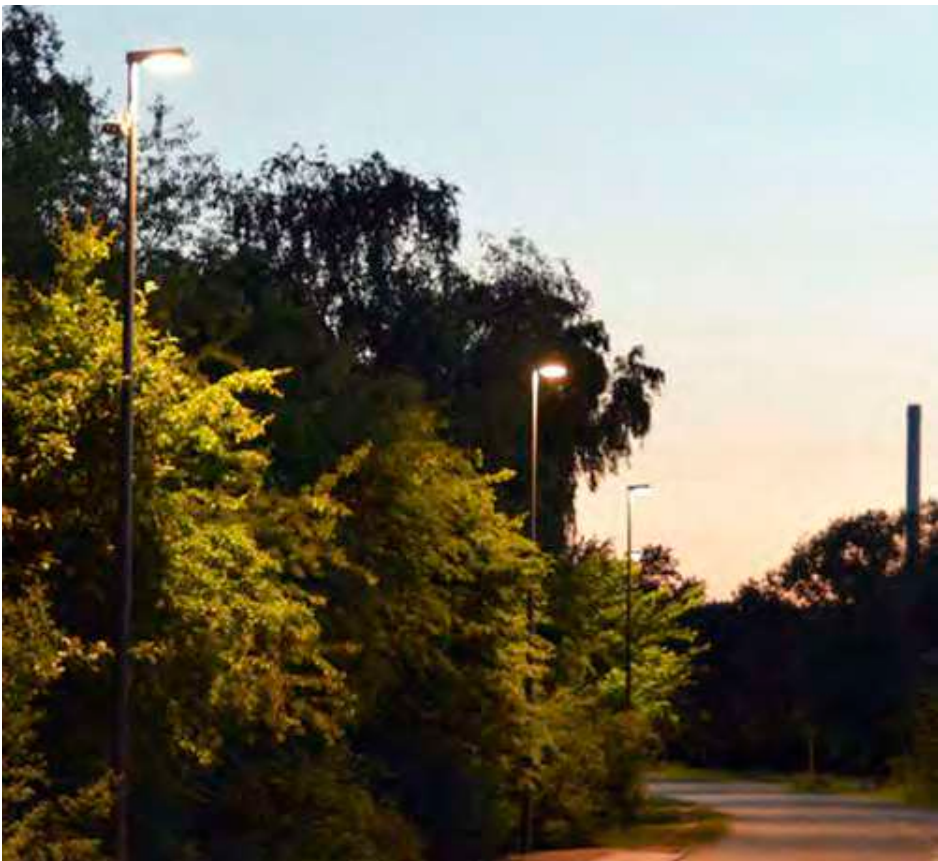
Column lighting to highways
