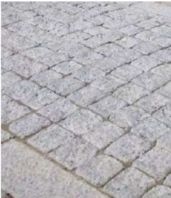
PAVING TYPE 3 - CONCRETE SETTS
