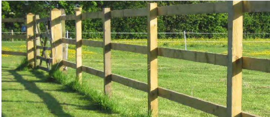
1.5m high timber post and rail fence
