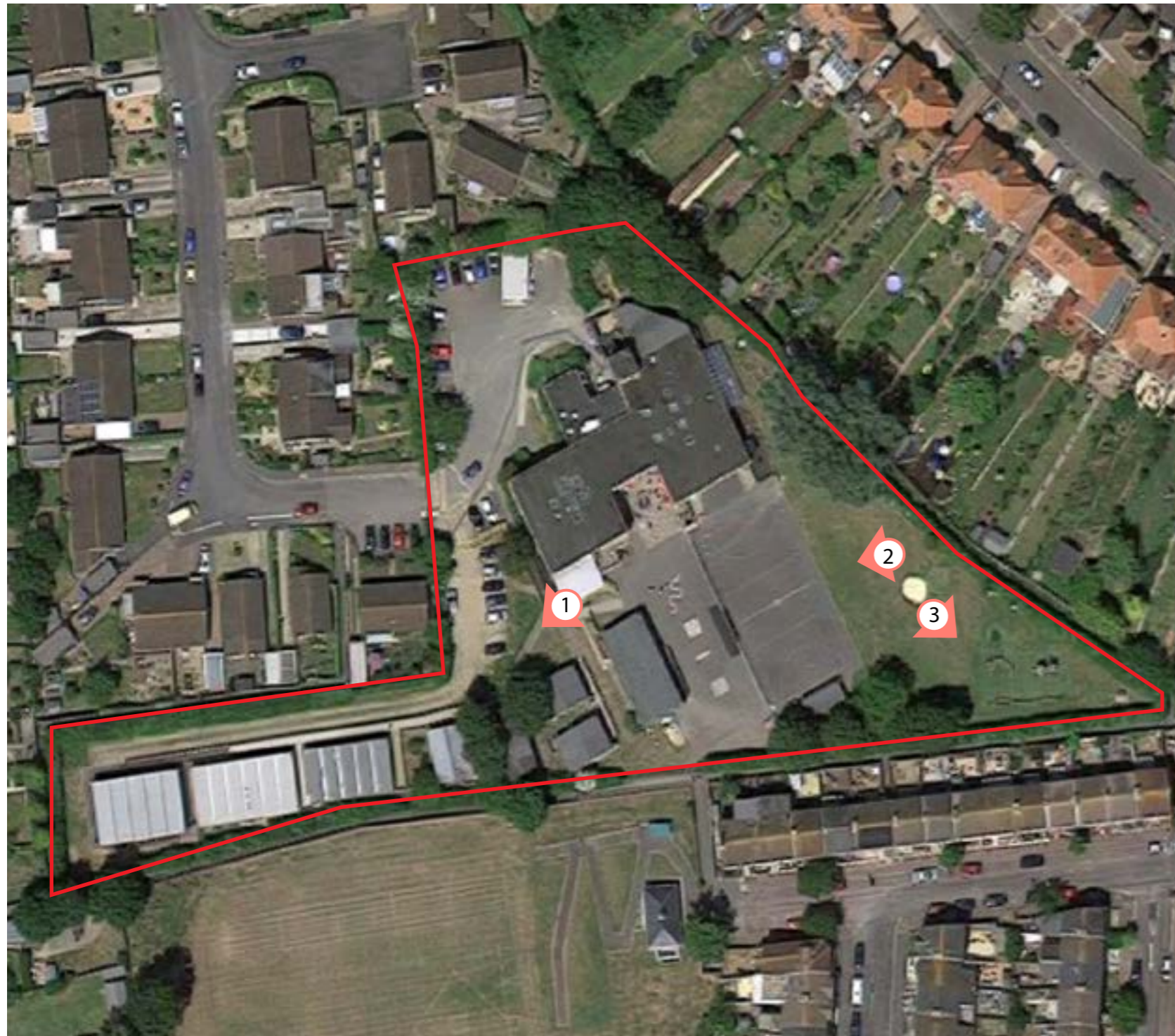
Aerial photographs showing the site on Highview School, Moat Farm Road, Folkestone
