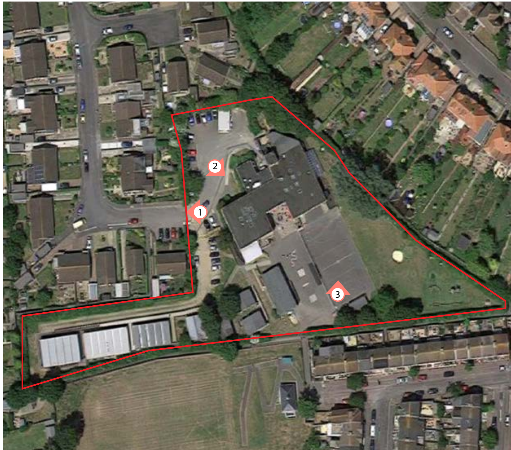
Aerial photographs showing the site on Highview School, Moat Farm Road, Folkestone
