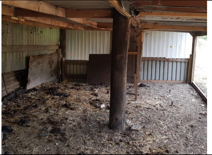
Photograph 7: Interior of B3.
