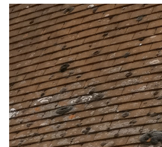
Image 2 - Existing roof tiles
