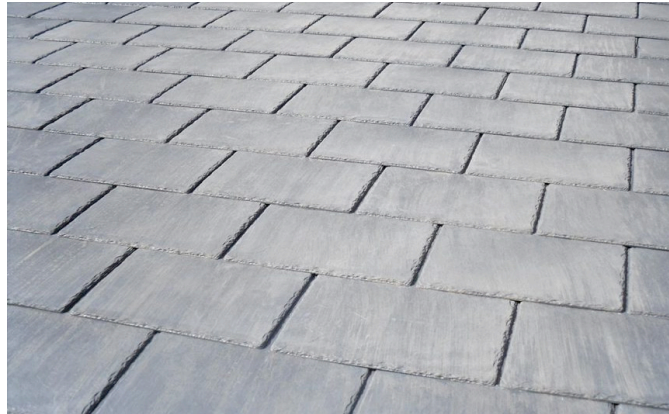
FIG 10- SLATE TILE ROOF.
