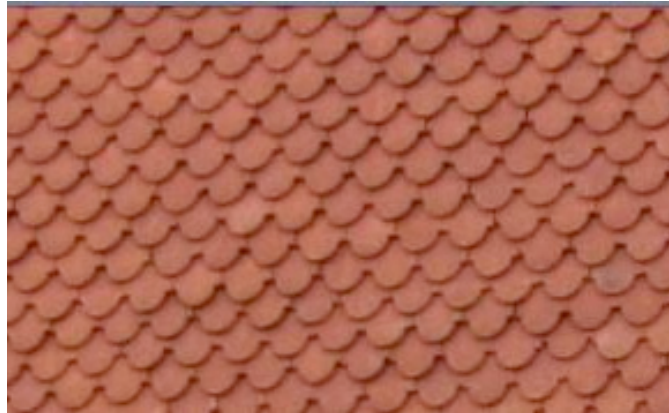
FIG 12- SPADE VERTICAL HANGING TILE
