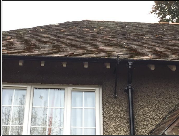
Photograph 14: Lifted clay tiles on the northern façade of the existing residential dwelling.
