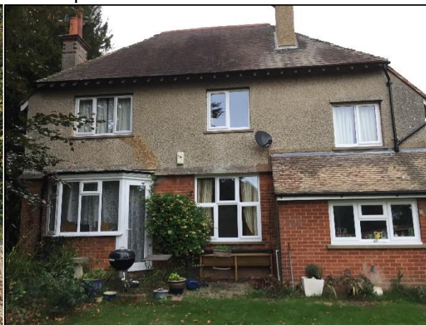
Photograph 12: The rear of the existing residential dwelling.
