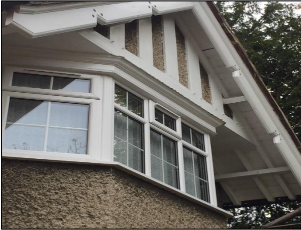
Photograph 13: Gaps within the soffit boards on the northern front of the residential dwelling.
