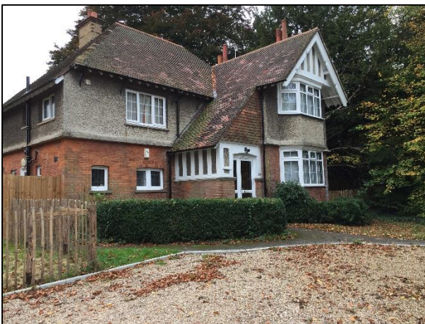
Photograph 11: The northern façade of the existing residential building.
