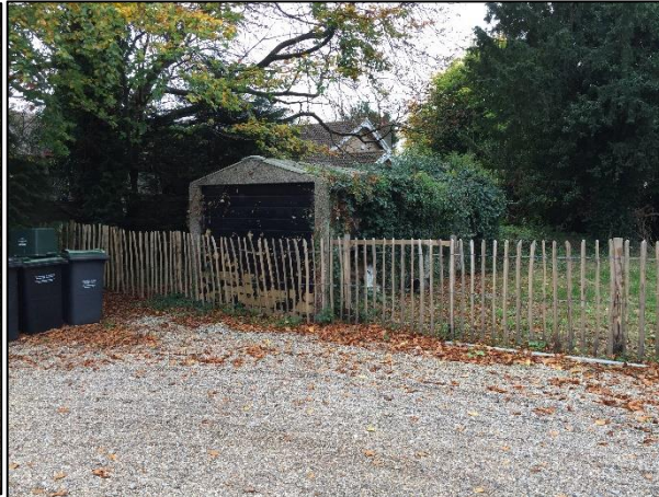
Photograph 4: Built structures on site with wooden fencing to the north of the development area.
