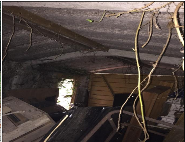
Photograph 16: Interior of the single-storey garage.
