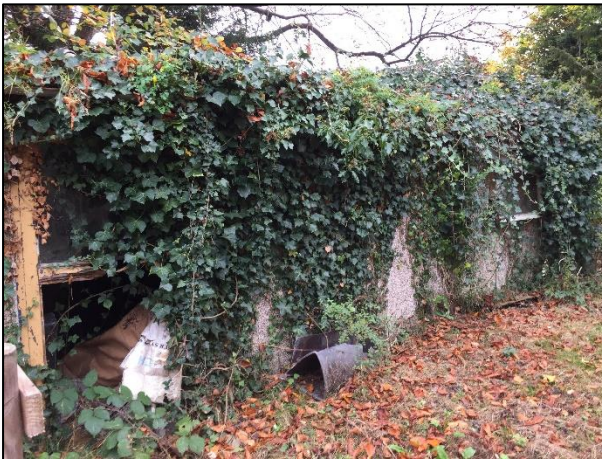
Photograph 17: Western façade of the single-storey garage with ivy coverings.
