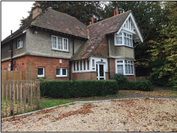
Photograph 3: Area of hardstanding comprising gravel drive and tarmac pedestrian path to the front of the existing residential dwelling.
