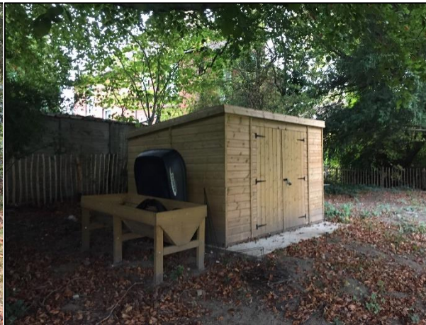
Photograph 18: Wooden garden shed located within the rear garden of the existing residential dwelling.
