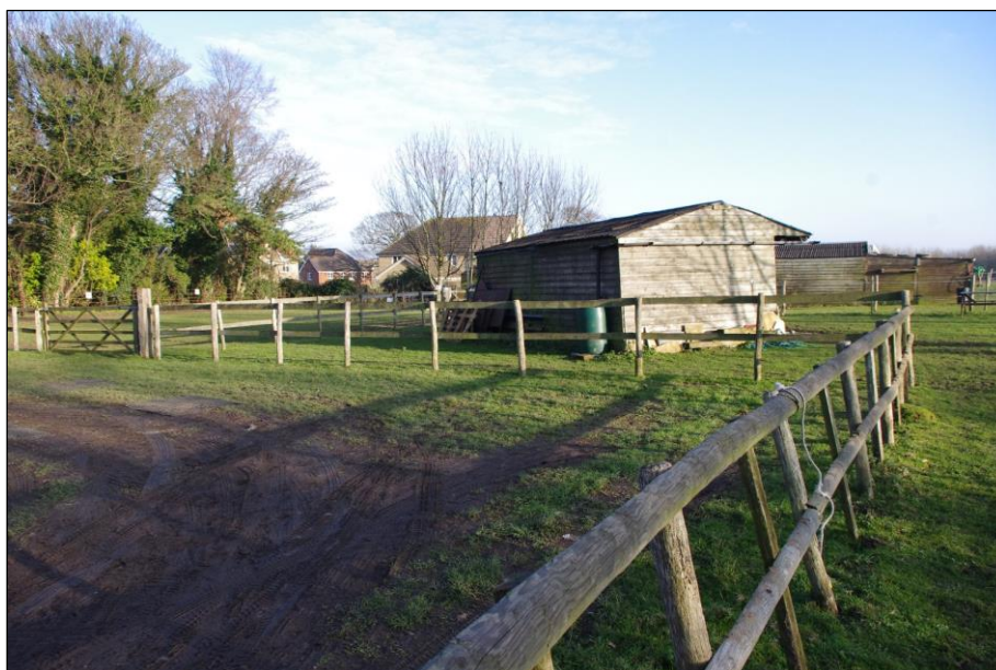
Plate 4.3: View looking east from the Site boundary access point off Dover Road. The Site contains modern outbuildings that are of no architectural or historic interest.
