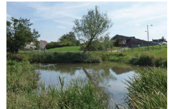
Typical Image: Attenuation pond and wetland planting
